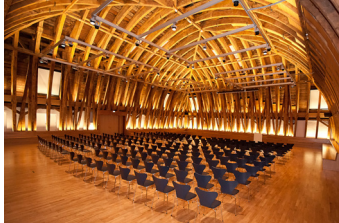
Cupola hall at TU Wien, serving as main lecture room © TU Wien
